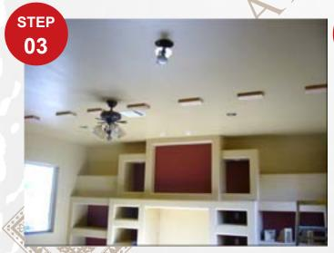
Apply 2x blocking with urethane adhesive and screws.
