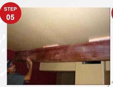
Cut beam to size and "Dry Fit" into place before attaching with glue and nails.
