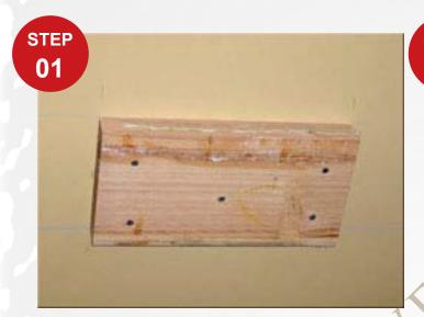
Layout spacing and chalk or pencil a straight line of were beams will go. make sure the line is referenced for the inside of the beam.
