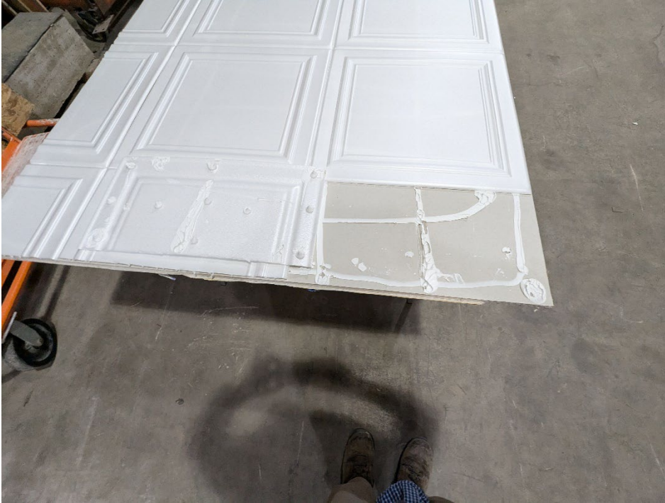
Figure 3 – Gypsum board (1 of 2) with specimen tiles partially installed
